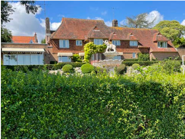
Rear elevation overlooking Clays Field
